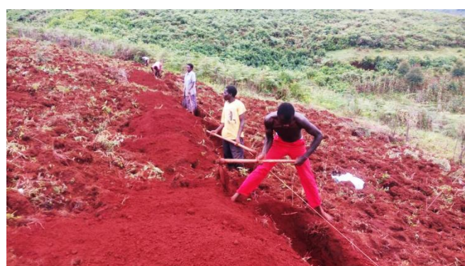
Figure 2: Constructing trenches along the slope to trap soil erosion is labor intensive in Mt. Elgon region. Photo: Bonny Woniala, 2018.
